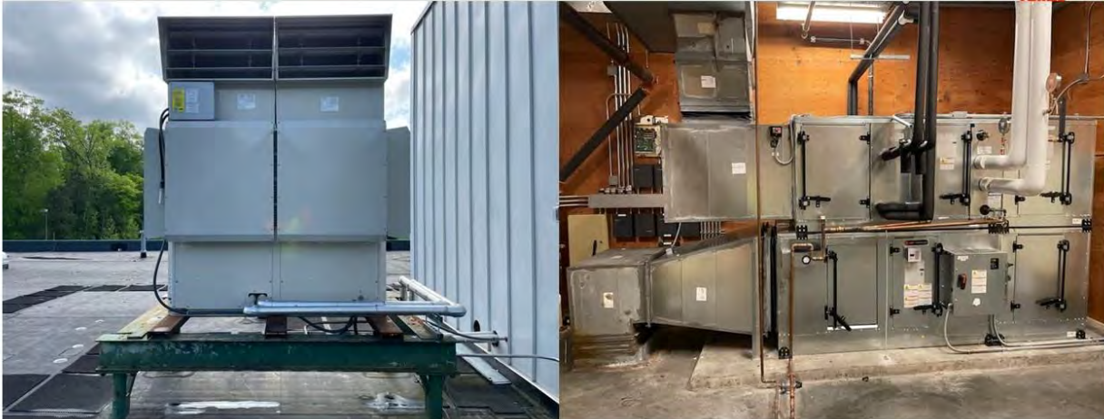
New split system serving the Artifact storage area
