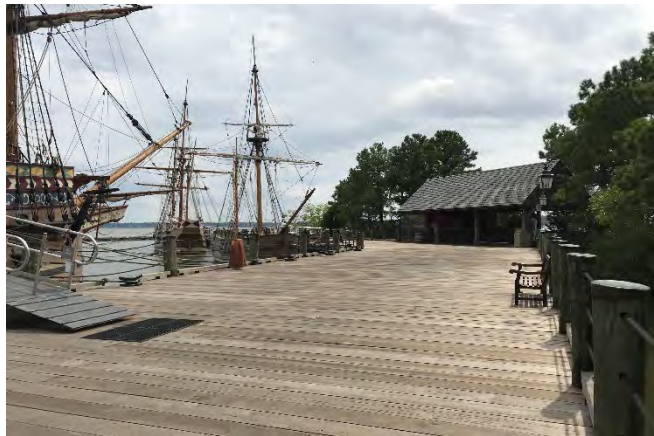
Figure 1: Phase I of the pier resulted in structural repairs and a complete replacement of the pier decking. The new structure and decking should extend the useful life of the pier by twenty years.
