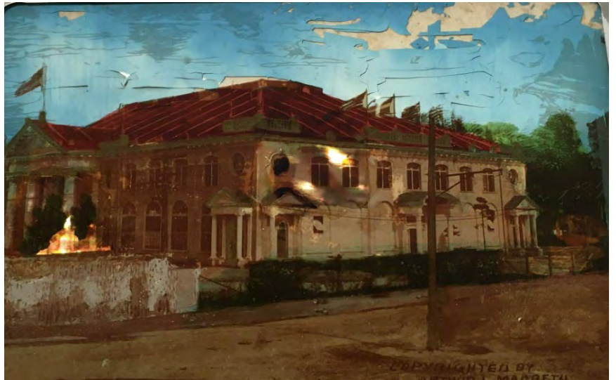
Macbeth, Arthur. Negro Building Jamestown Exposition 1907 . Photograph on glass plate. Jamestown-Yorktown Foundation
